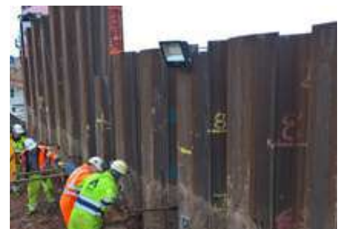
AWPR Sheet Pile Wall
