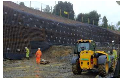
Soil Nailing at Mill Timber
